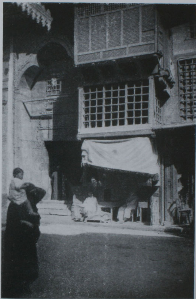
CAIRO: TYPICAL NATIVE HOUSE
