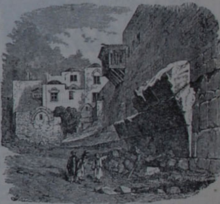
No. 1.—Remains of Arch of Bridge. (S.W. angle of Haram.)
